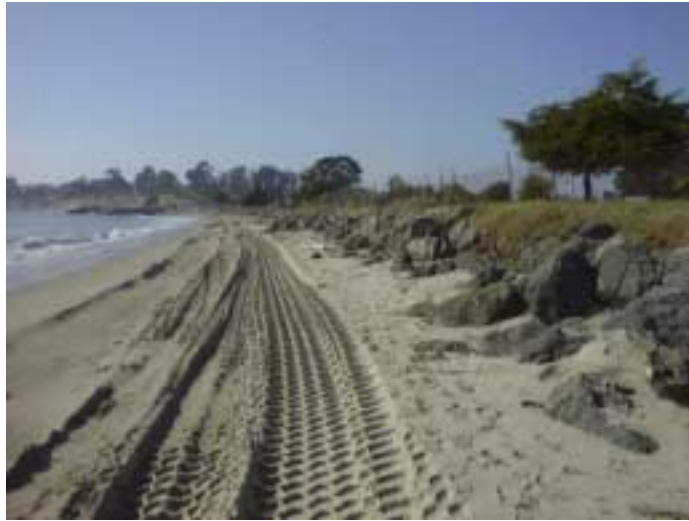
Figure 5. Seawall in front of Goleta Beach County Park, looking west. [Photo: Shawn Kelly, November 30]
